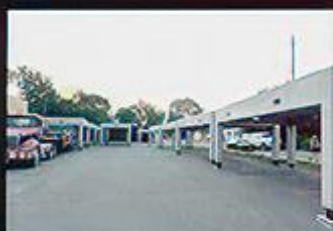
Precast Structural Building Units are staged at / near the construction site in advance of construction.
